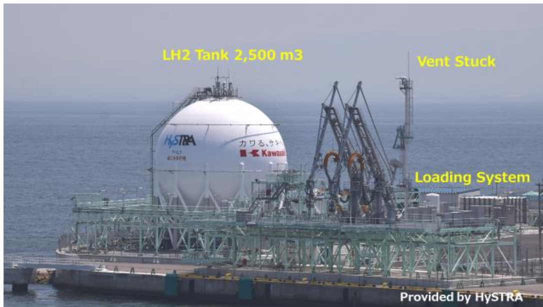
Figure 4.16: Status of Construction of LH2 Cargo Loading Base (Kobe Airport Island) in April 2020
