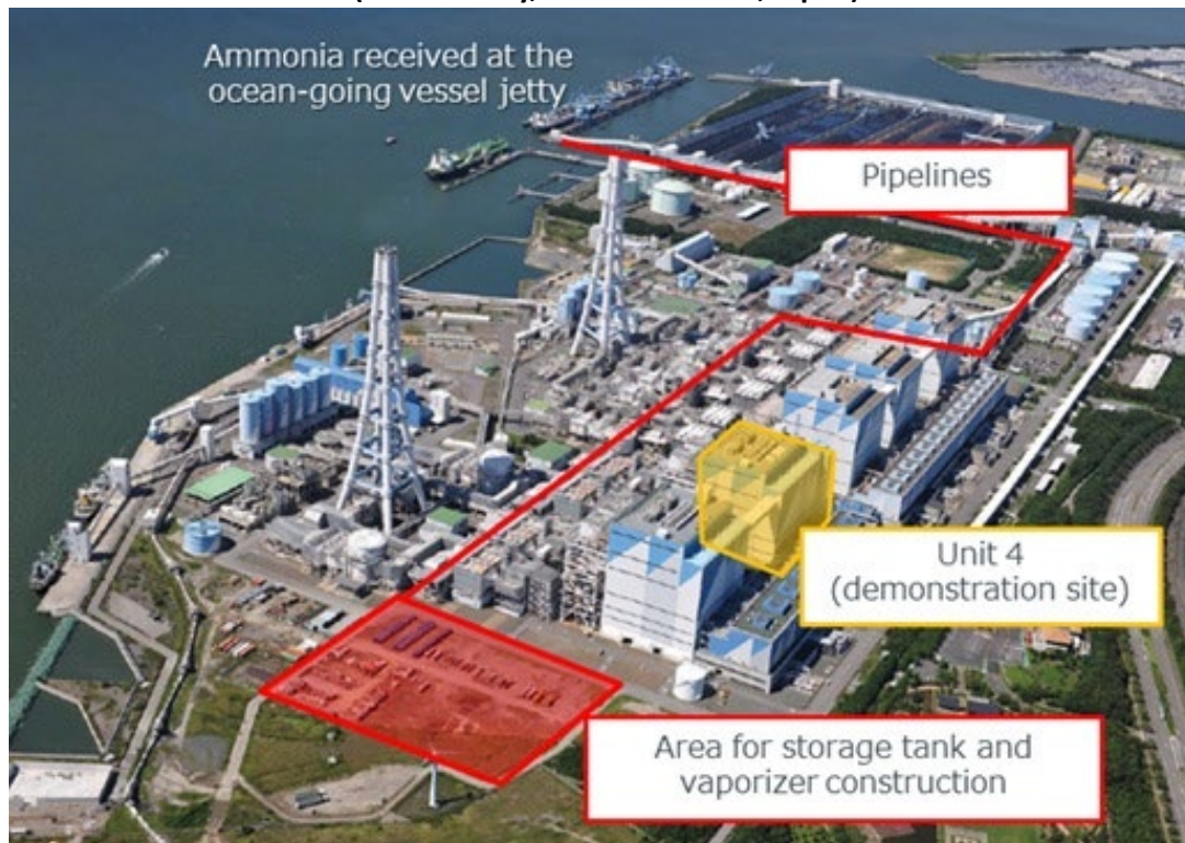
Figure 4.2. Project Site at the Hekinan Thermal Power Station (Hekinan City, Aichi Prefecture, Japan)
