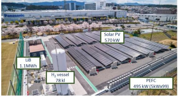
Figure 2.13. Demonstration of RE100 Factory, Panasonic 'H<sub>2</sub> Kibou Field Demonstration'
