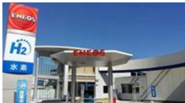
Figure 3.26. ENEOS Yokohama Tsunashima Hydrogen Station
