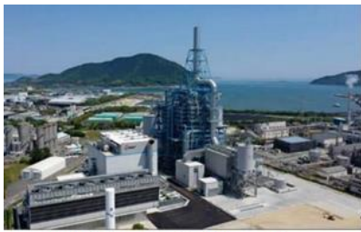
Hofu Biomass Co-firing unit (Source : Chugoku Electric Power Co.)
