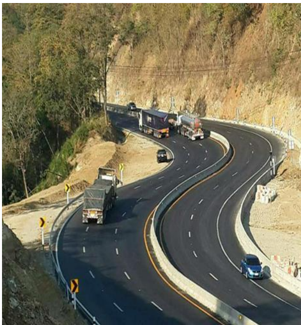
Figure 5: Highway Linking Ta to Mae Sot
