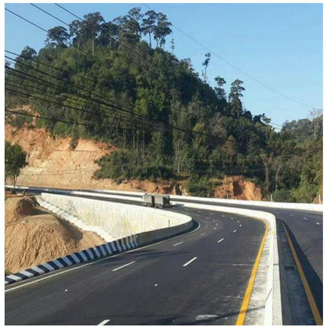
Figure 6: Highway Linking Ta to Mae Sot
