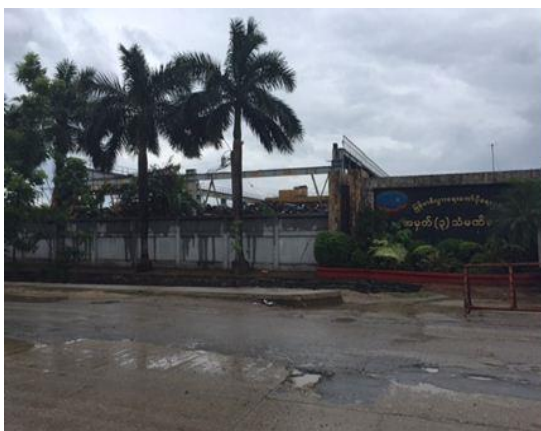
Figure 51. Steel plant of MEC at Yangon
