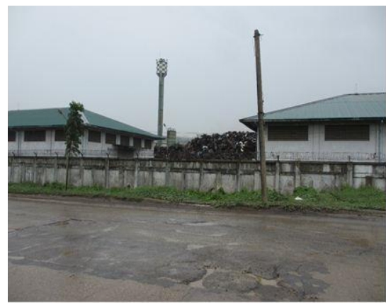
Figure 52. Steel plant of MEC at Yangon
