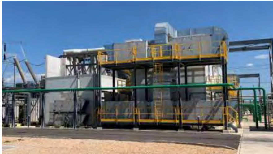
Figure 0.7. Synchronous Condenser Systems Installed in Italy
