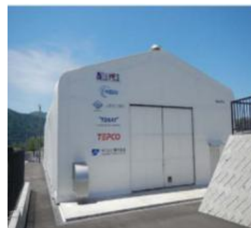
P2G experimental research building exterior
