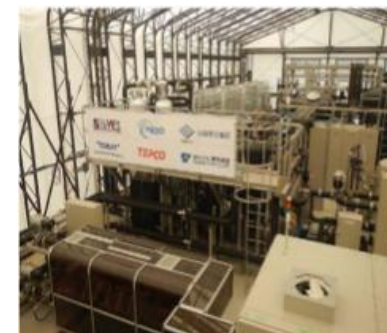
Inside the P2G experimental research building
