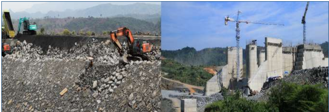
Figure 3.54. Construction of the Jatigede Dam
