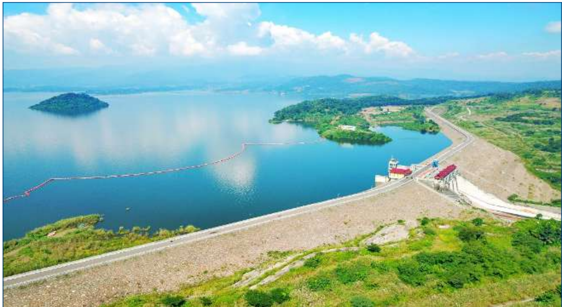
Figure 3.57. Jatigede Dam and Reservoir
