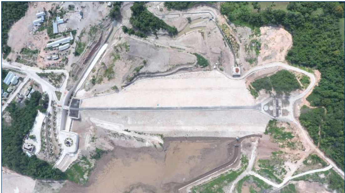
Figure 3.58. Raknamo Dam Development
