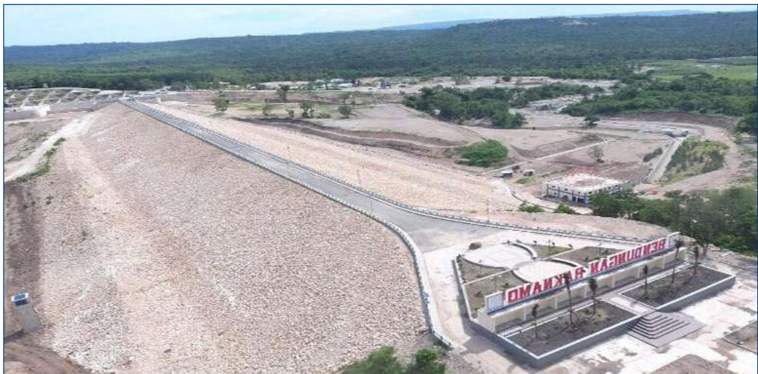
Figure 3.59. The Area around the Raknamo Dam
