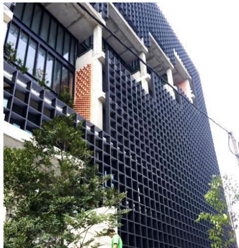
Figure 1: Egg-Crate Louvres Design
