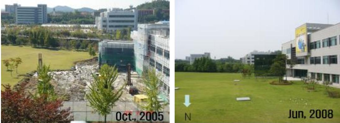
Note: During the installation of borehole heat exchangers (BHEs) (left) and after covering BHEs with green grasses (right).
