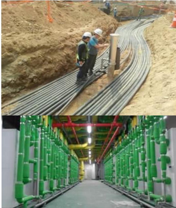
Note: From top, drilling of borehole for BHE, trench line of heat exchanger pipes into building, and heat pumps in the basement floor of building.
