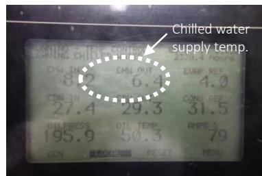
Operation panel of chiller.
