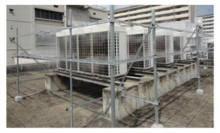
Figure 2-49. Spraying Mist on Compressor Units
