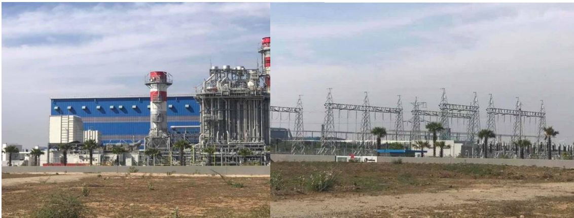
Figure 3.9: Myingyan Power Plant
