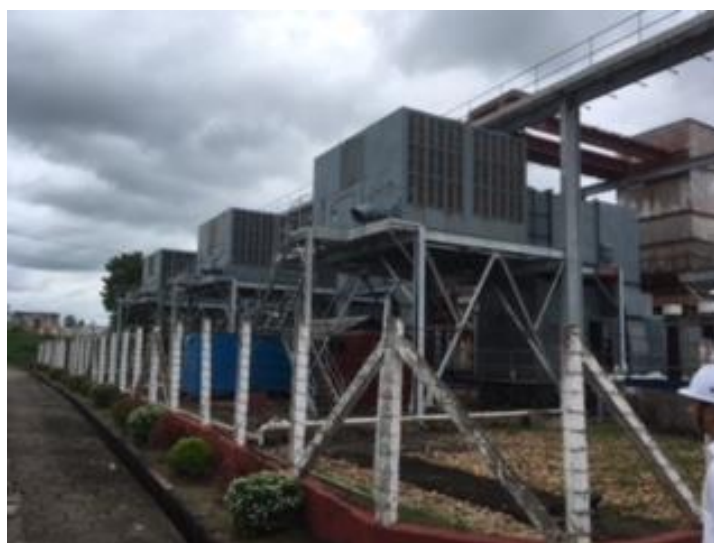
Figure 6.3: Shwedaung Gas-Turbine Power Plant
