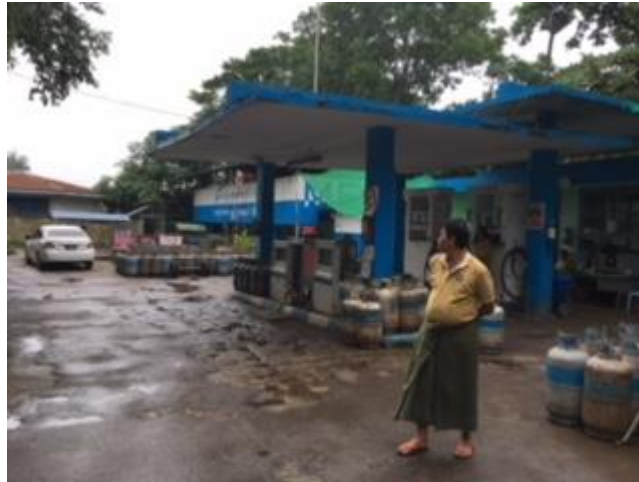
Figure 5.8: Liquefied Petroleum Gas Supply Station in Yangon City
