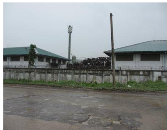
Figure 52. Steel plant of MEC at Yangon
