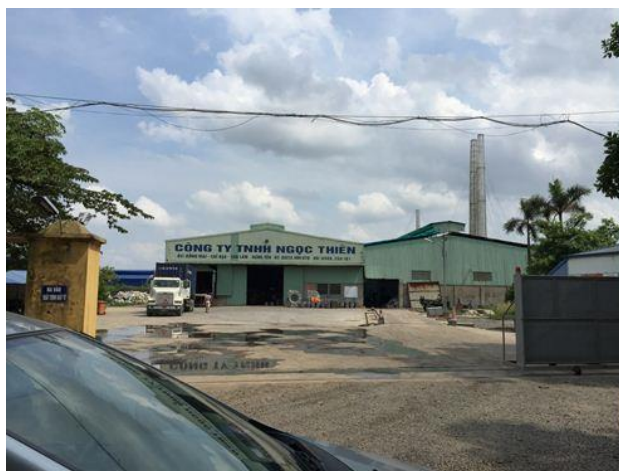
Figure 110. Battery and lead recycling company
