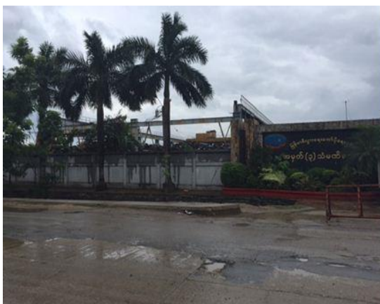
Figure 51. Steel plant of MEC at Yangon
