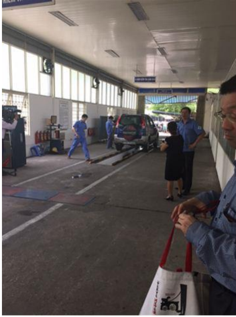
Figure 116. Car inspection facility
