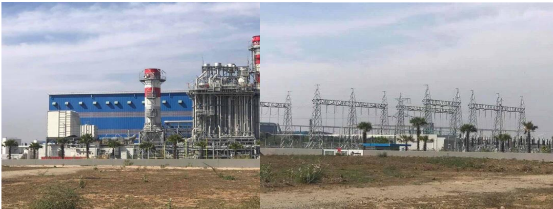
Figure 3.9: Myingyan Power Plant
