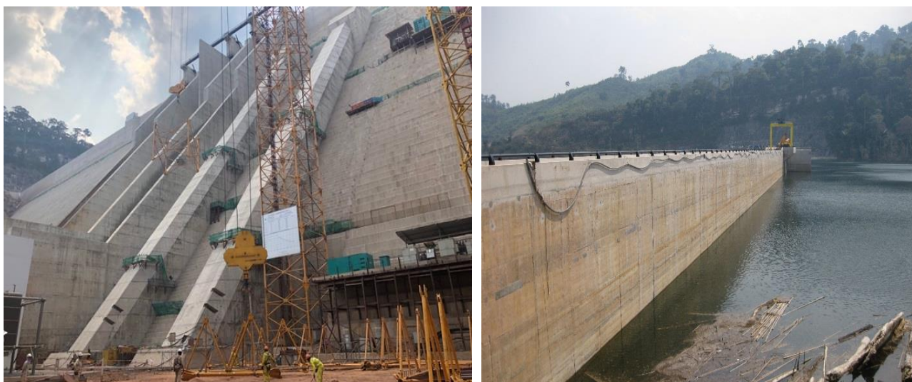
Figure 3.5: Nam Ngeip 1 Hydropower Dam Site
