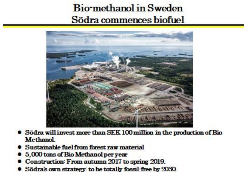
Figure 4.3.7. Södra Biomethanol Plant in Sweden
