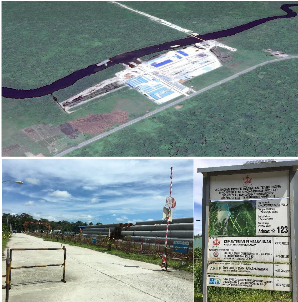
Figure 6.2: Condition of Gate Zone
