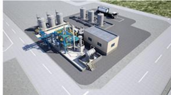
Dehydrogenation plant in the coastal area of Kawasaki
