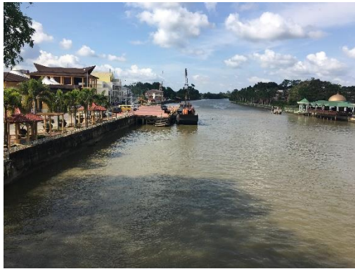
View from the Jalan Labu Bridge (downstream)
