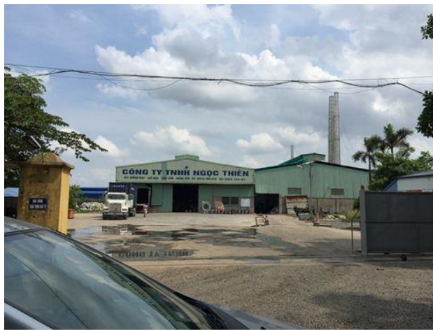
Figure 110. Battery and lead recycling company
