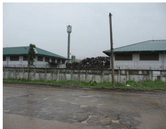
Figure 52. Steel plant of MEC at Yangon
