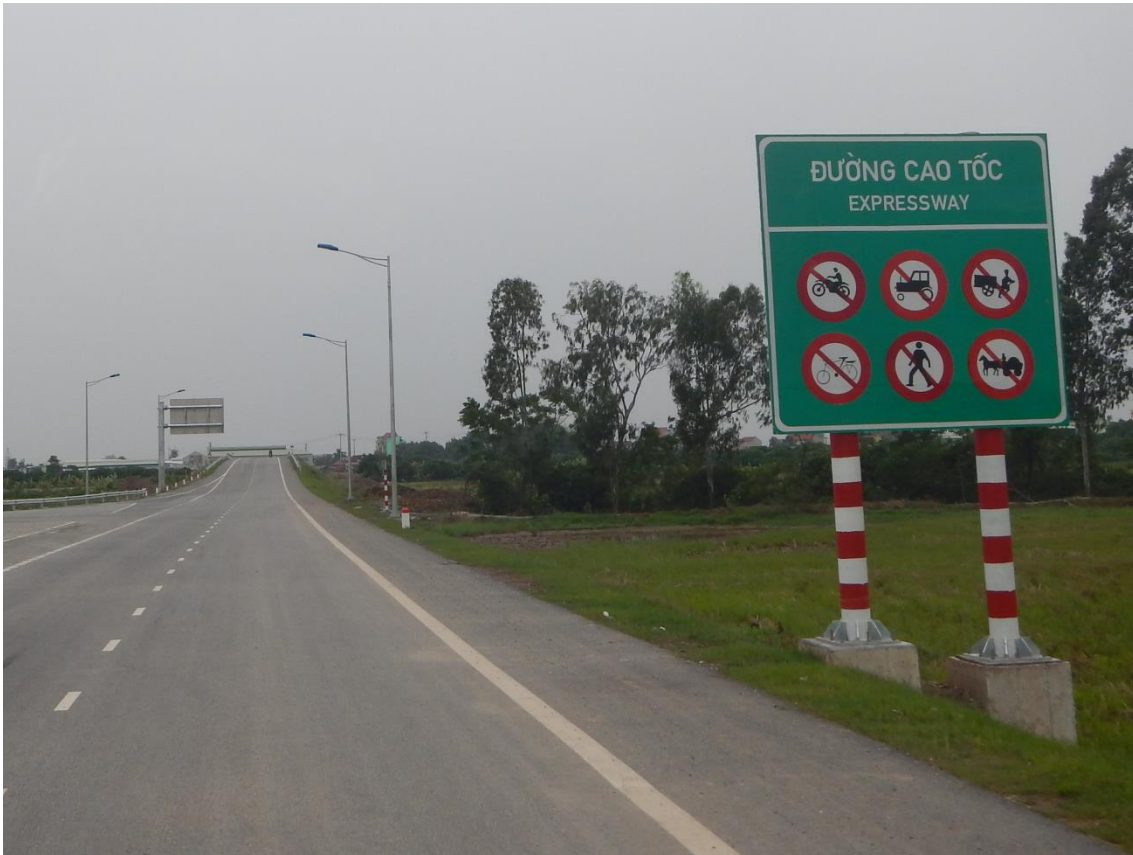
Figure 6.2. Example of a Road Sign at the Entrance of the Hanoi–Hai Phong Expressway
