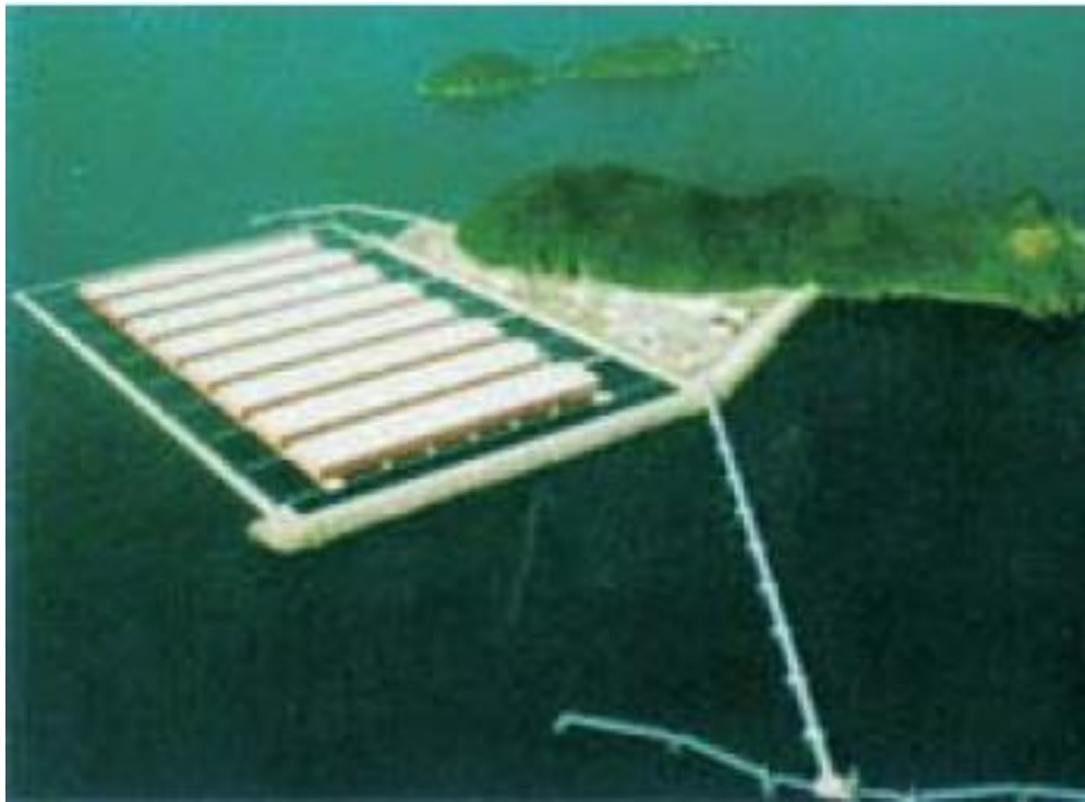
Figure 2-2: Shirashima Stockpiling Base
