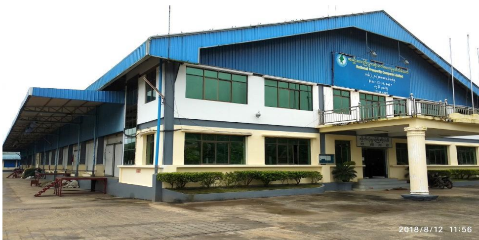
Figure 6.29: National Prosperity's Cold Store Facility in Muse
