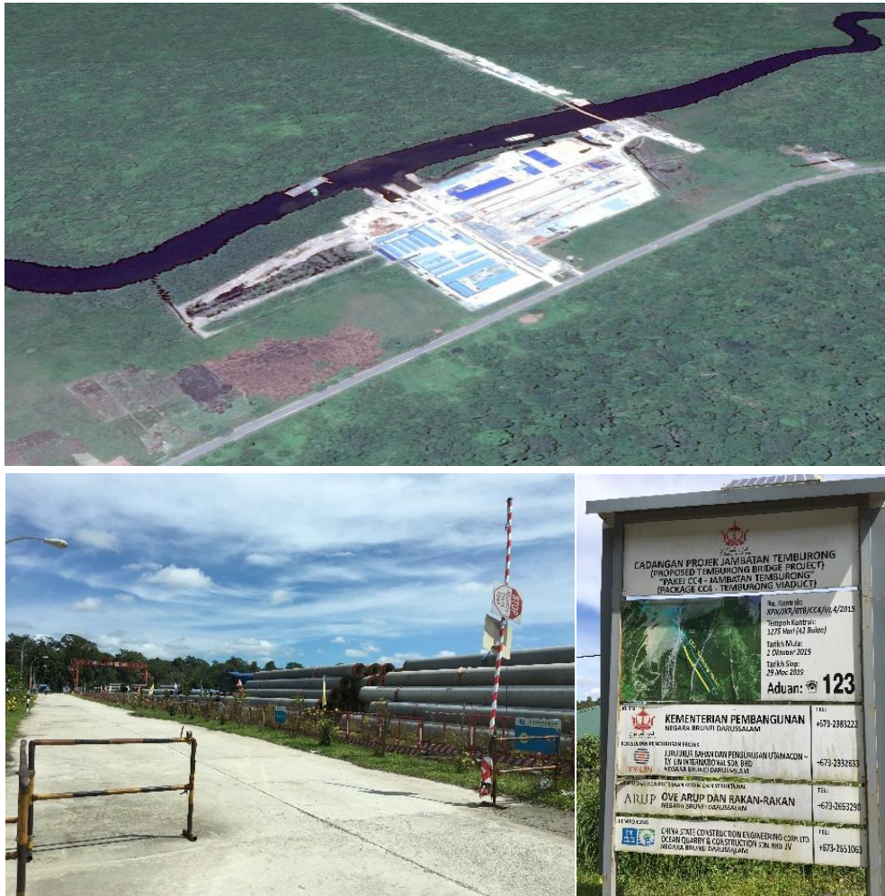
Figure 6.2: Condition of Gate Zone
