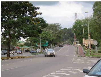
Jalan Labu Bridge
