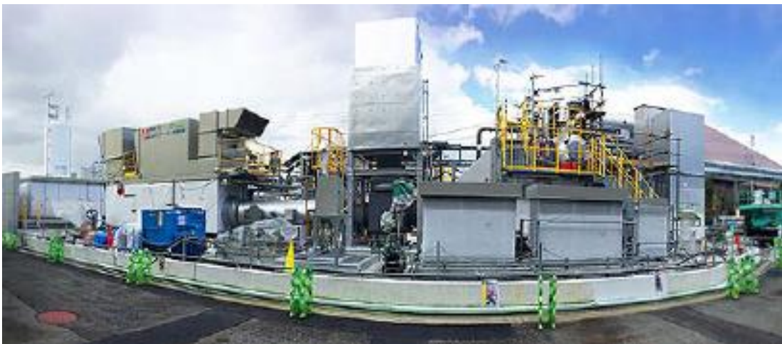
Figure 5.6: Hydrogen Production and Supply Facility
