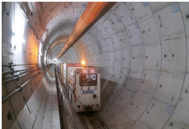
Graphic 11. Jakarta MRT Construction Site (2016)
