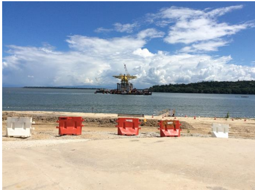
Graphic 10. Temburong Bridge Construction Site, Brunei Darussalam (2016)
