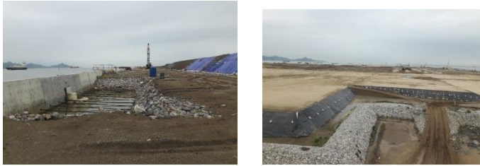
Graphic 9. Lack Huyen Port Construction Site (2016)
