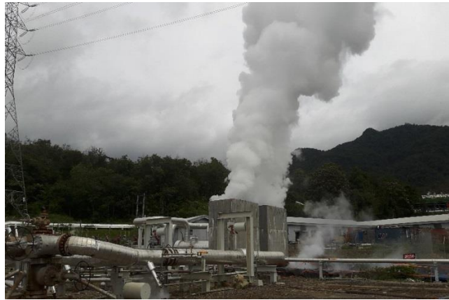
Graphic 3. Sarulla Geothermal Power Plant
