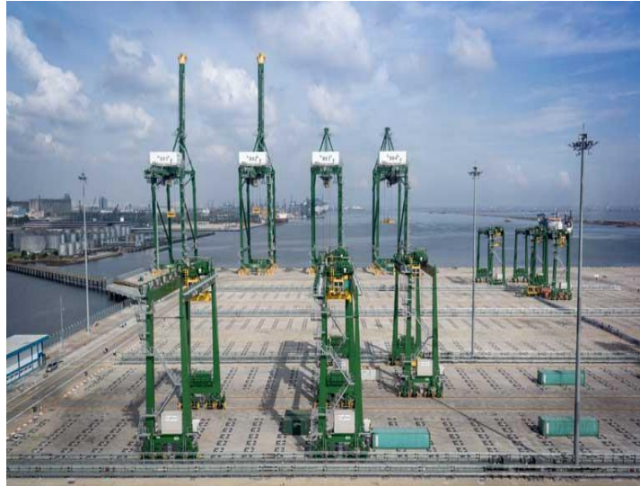
CT1, new container terminal
