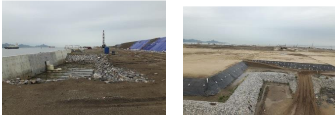
Graphic 9. Lack Huyen Port Construction Site (2016)
