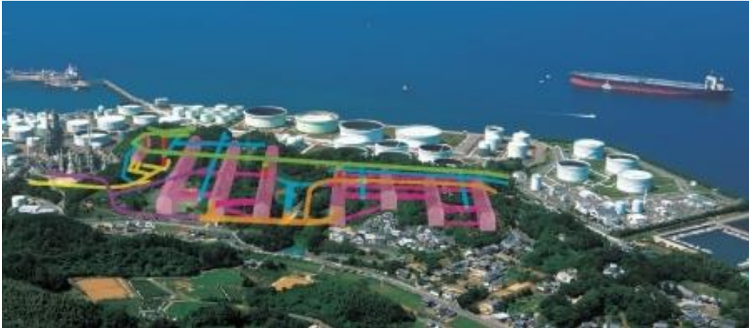
Figure 2-2. Image of an Underground Stockpiling Base
