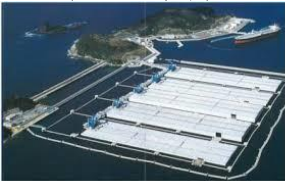
Figure 2-5. View of a Floating Stockpiling Base
