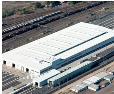
Figure 12.3. The Auburn Maintenance Centre
