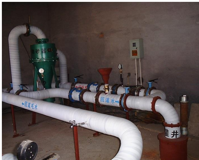
Figure 4.1-B5. Installation of Geothermal Reinjection Well in Xiaotangshan Field
