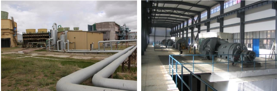
Figure 4.1-A3. Yangbajain Geothermal Power Station, Outdoor View (left) and Indoor View (right)
