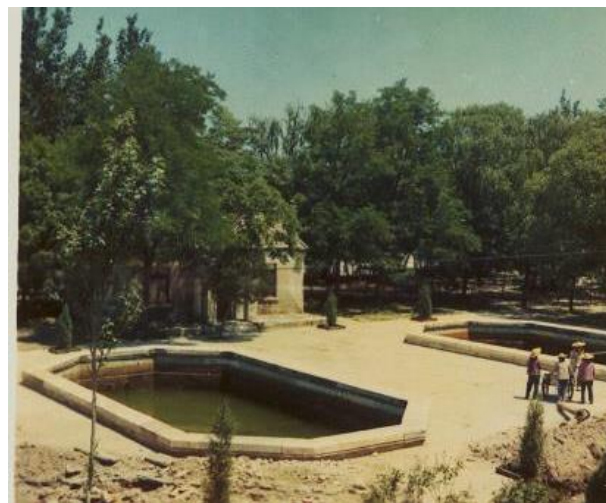
Figure 4.1-B2. Lower Water Level of the Eastern Spring (right) and the Western Spring (left) in Xiaotangshan Hot Spring Sanatorium
