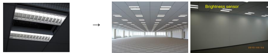
Typical fluorescent lighting fixture
