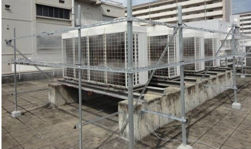
Figure 2-49. Spraying Mist on Compressor Units
