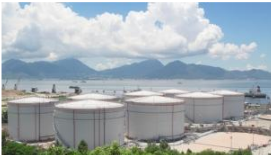
Figure A-1-5. Storage Tanks at the CNPC’s Fuel Terminal in Kyaukphyu
