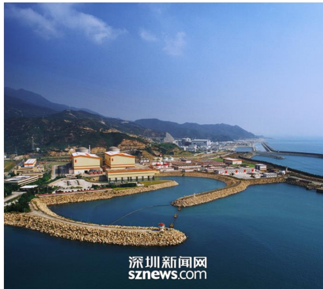
Figure 2.19 Daya Bay Nuclear Power Station (front) and Ling Ao Nuclear Power Station(back)
