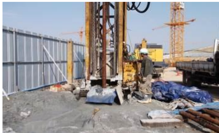
Figure 5.3-2. Ground Source Heat Pumps for the Government Building Complex, Sejong Metropolitan City
