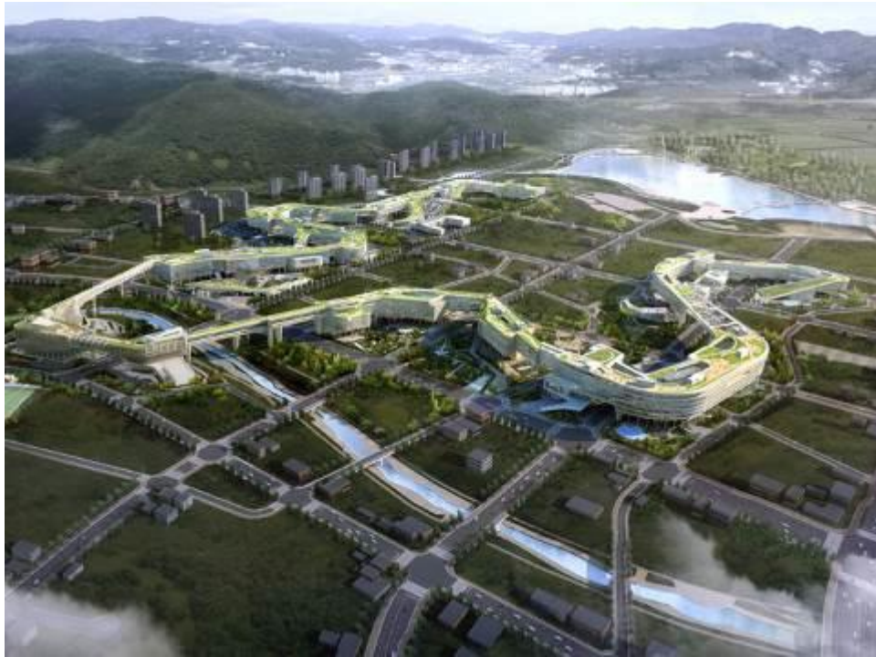
Figure 5.3-1. Bird's-eye View of Zones 1 and 2 of the Government Building Complex, Sejong Metropolitan City
