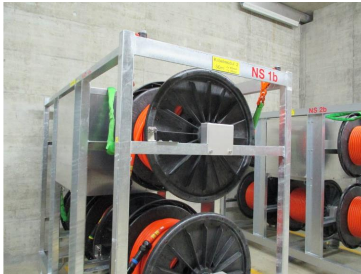
Figure 3-1-1. A Cable Module Set in the External Storage Centre for Emergency Equipment
