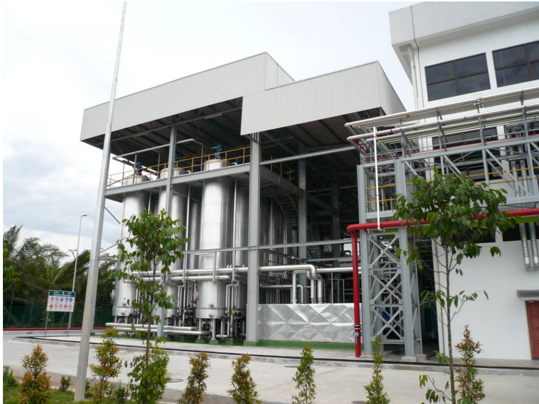
Figure 38 Palm biodiesel winterization plant at Sime Darby Biodiesel Sdn. Bhd., Malaysia.
